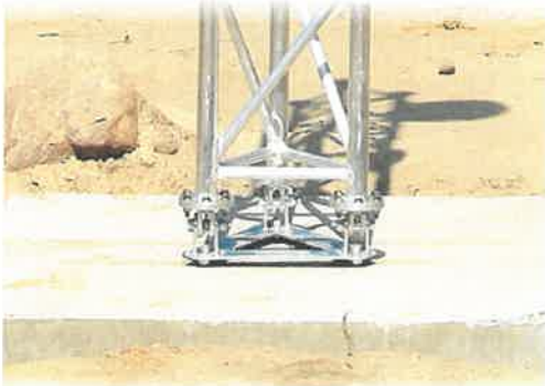
A ready foundation with the MK tower in place
